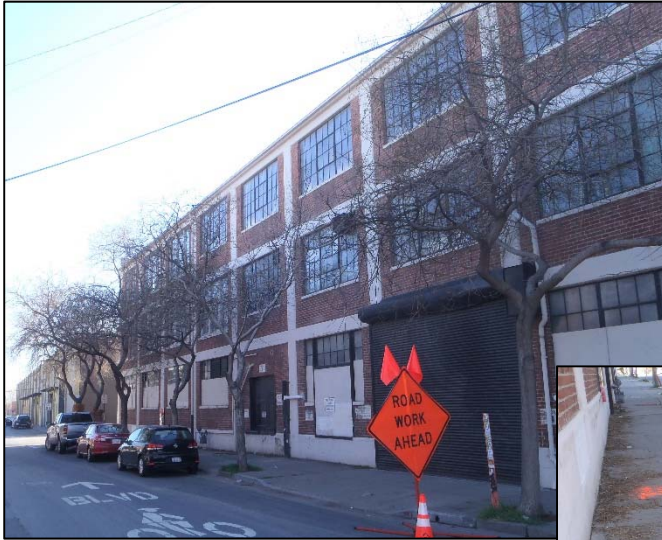
Photo 1 (L): Looking southwest at Japanese pagoda trees #6-11 (R to L). Condition was variable but almost all had displaced the surrounding sidewalk, curb and gutter from 2" to 8" (inset). Inset was taken at tree #11 looking northeast.
