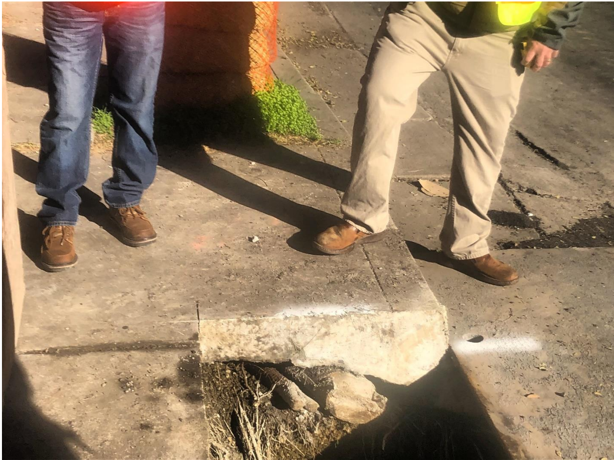
Photo 3. Photo left shows the 7" and 3" roots that were severed during hardscape removal.
