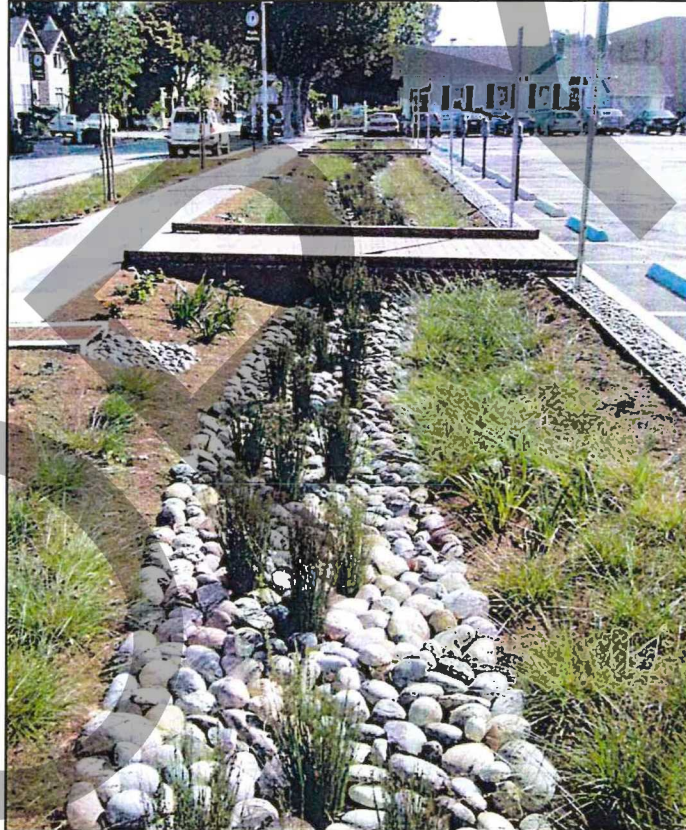
Figure C-5. Donnelly Street Green Street Project. The Donnelly Street Green Street Project includes a rain garden, pictured at right, which captures runoff from the adjacent commercial buildings and parking lot. The rain garden was designed with no underdrain and an enlarged subsurface layer of rock, which serves as a reservoir and allows runoff to slowly infiltrate to the underlying soil. The system was designed for onsite management of flows that exceed the 30-year storm. An overflow to the curb is provided for a 50- to 100-year event scenario. Source: City of Burlingame
