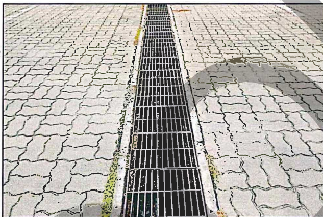
Figure C-7. Trench Drain. A trench drain can be used to convey runoff to GI facilities.
