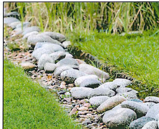
Figure C-8. Pervious Drainage Channel. Pervious, unlined drainage channels can be designed to convey runoff to GI facilities.
