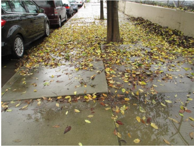
Photo 5. Photo shows the hackberry trees looking east with the smaller tree in the foreground. This tree has not thrived, likely due to a restrictive soil environment. There is also sidewalk uplift.
