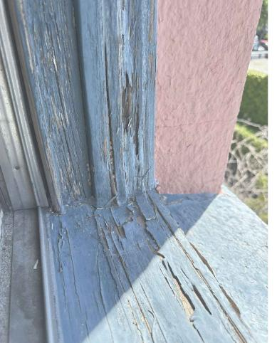
ERIOR CONDITION - SILLS AND JAMBS APPEAR TO LACEMENT. SASH SEEMS RESTORABLE AND DOUBLE NDOWS REMAIN WORKABLE.
