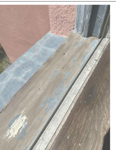
CONDITION ON THE EXTERIOR BUT INTERIOR IN GOOD DOUBLE HUNG WINDOWS WHERE OCCUR, WORK Y SMOOTHLY. EXTERIOR SANDING AND PATCHING MORE EFFORT THAN CONDITION A BUT SILLS AND RESTORABLE.
