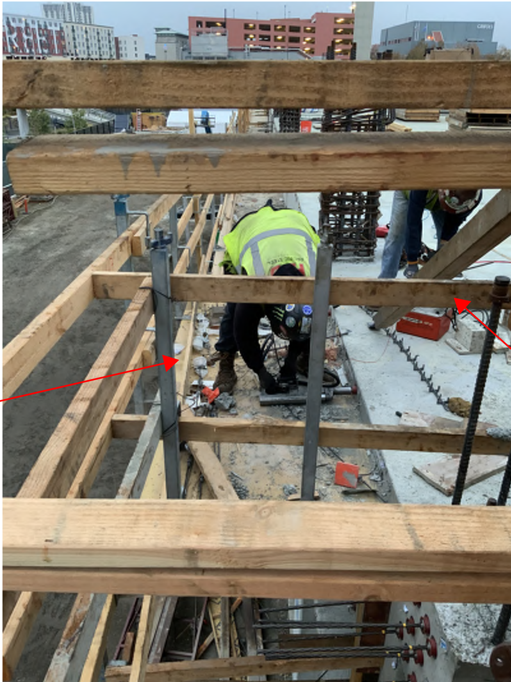
Exhibit 1: Typical "Stressing" activity. This activity is performed by a 3 man crew.
