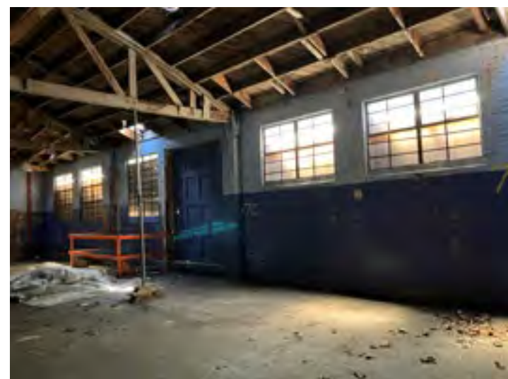
5. The door and windows along 40th Street remain.
