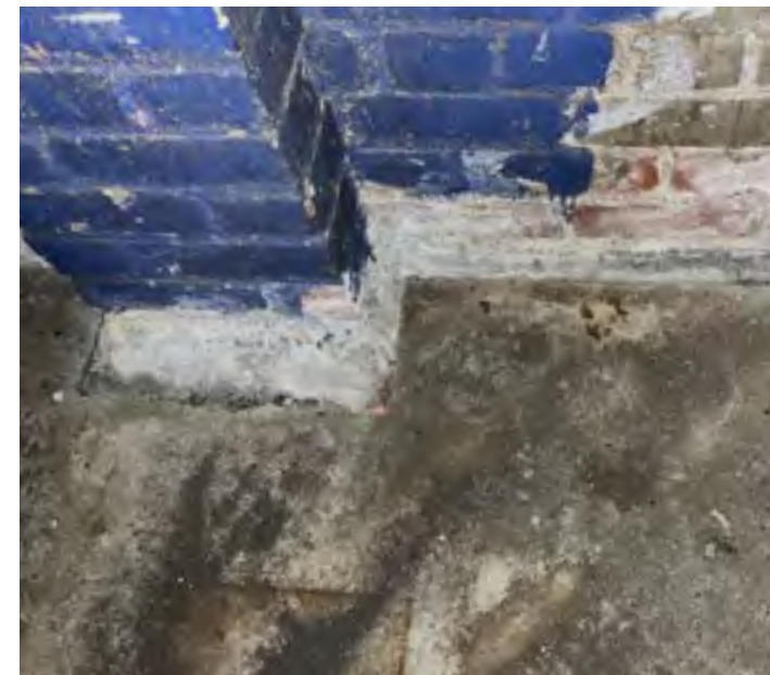
19. Concrete slab condition at perimeter brick wall.
