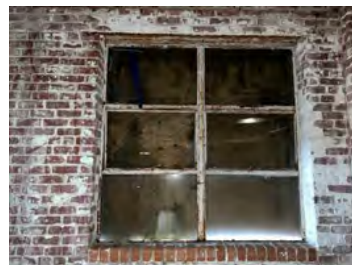
8. Interior view of Hollis Street window. The windows on this west facade remain and are boarded from the exterior.
