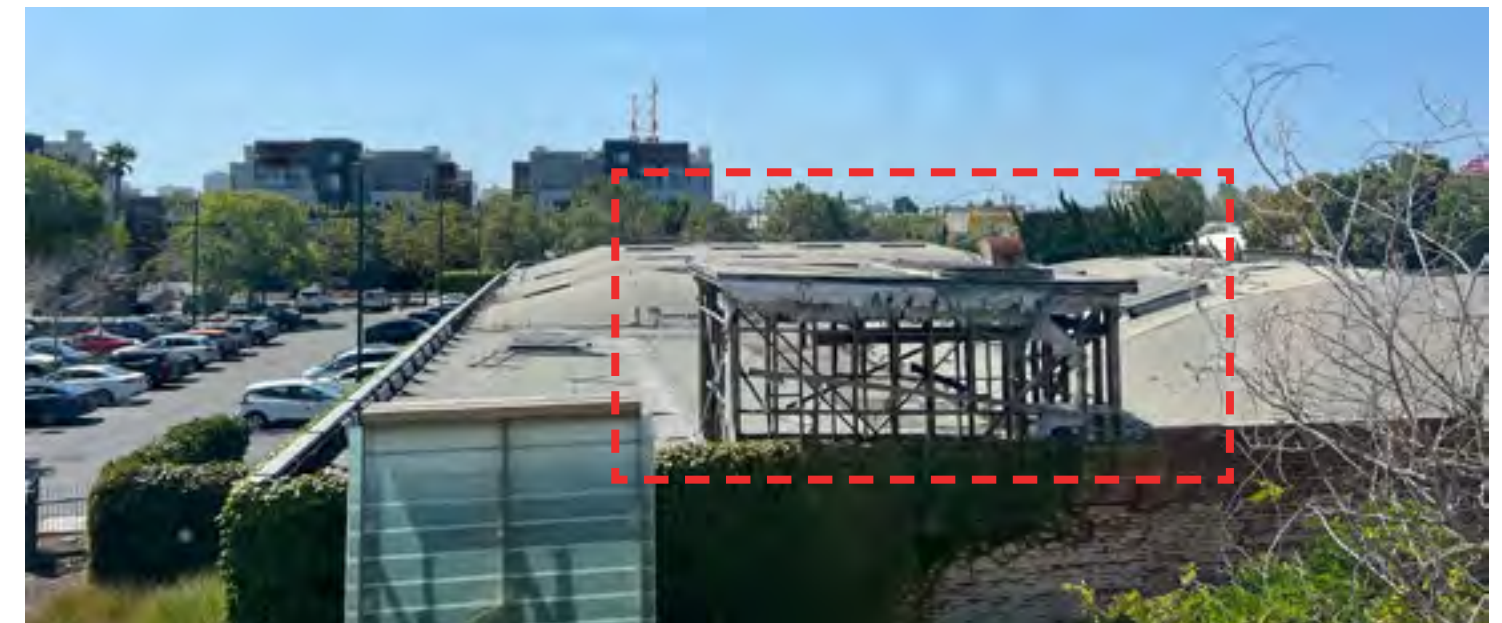
15. North roof view from upper level of adjacent Emeryville Civic Center.
