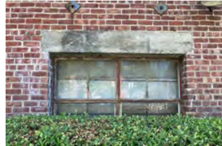
7. Example of existing west facade window with historic concrete lintel.
