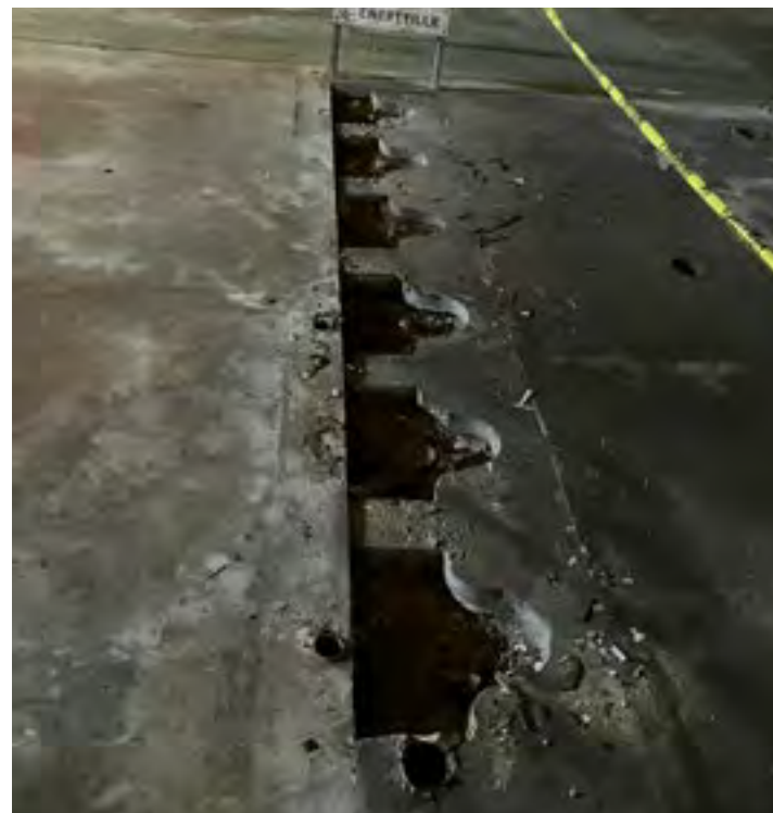
16. Slab condition from demolished restroom lavatories.
