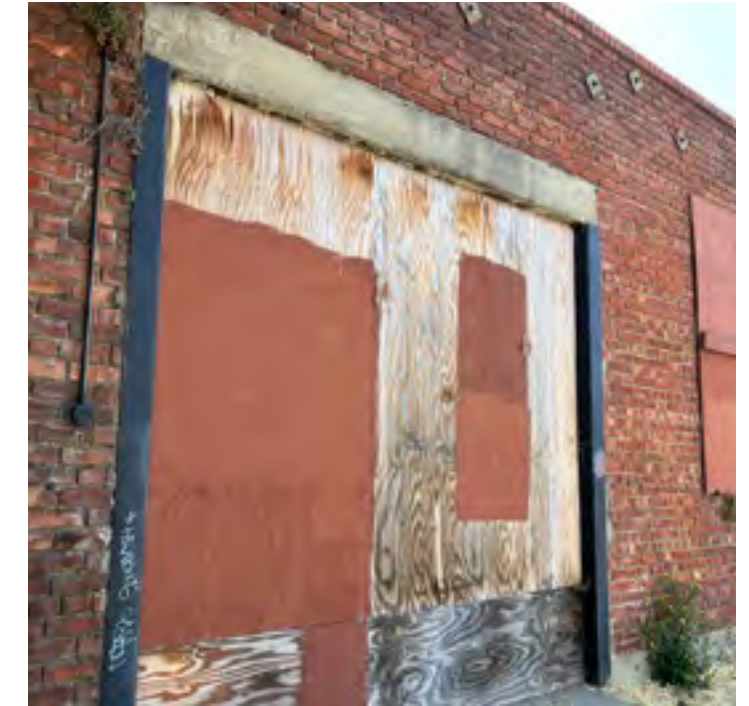
9. Previously demolished door with concrete lintel boarded up on Hollis Street.
