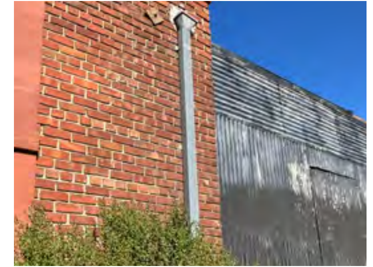
3. South brick facade meeting metal cladding.
