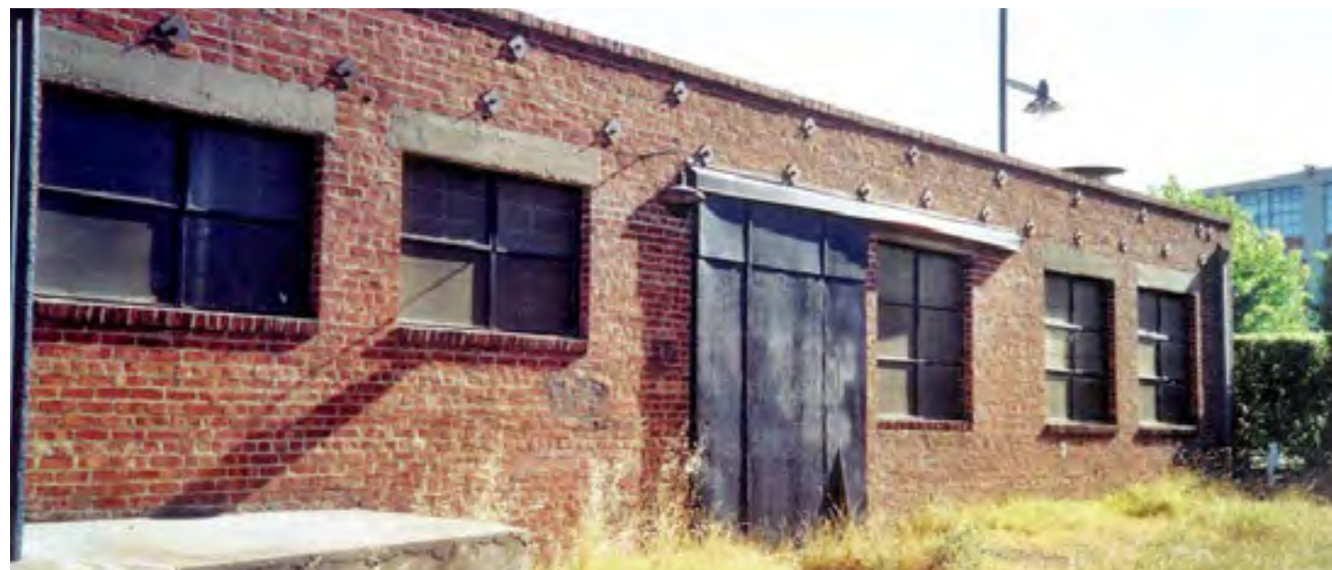
Historical character defining features depicted including brick facade, concrete lintels and horizontal repeating elements | image source: Emeryville Historical Society (EHS) Photo Archive
