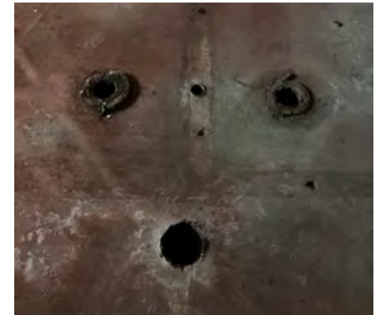
20. Existing holes in concrete slab from demolished toilets.
