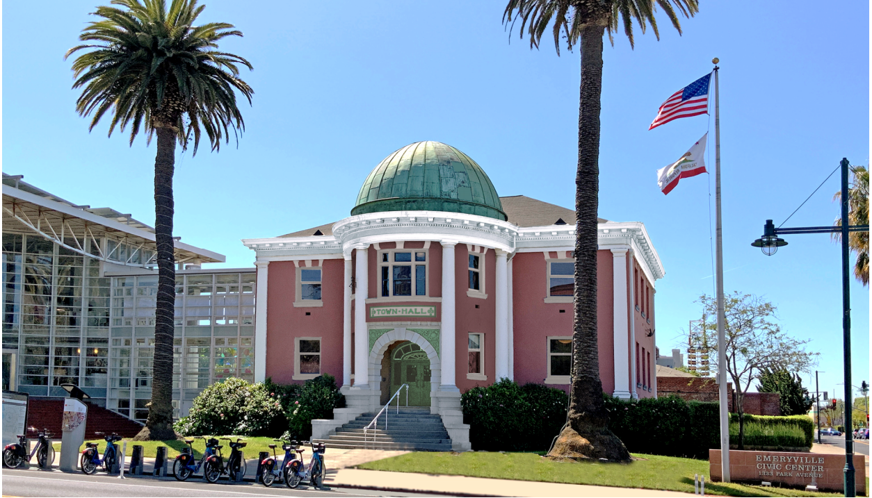
CITY OF EMERYVILLE OLD AND NEW CITY HALL EXTERIOR PAINTING
